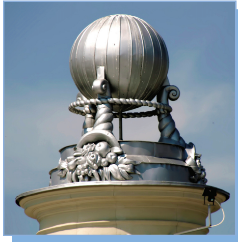
The dome above the Main Entrance
