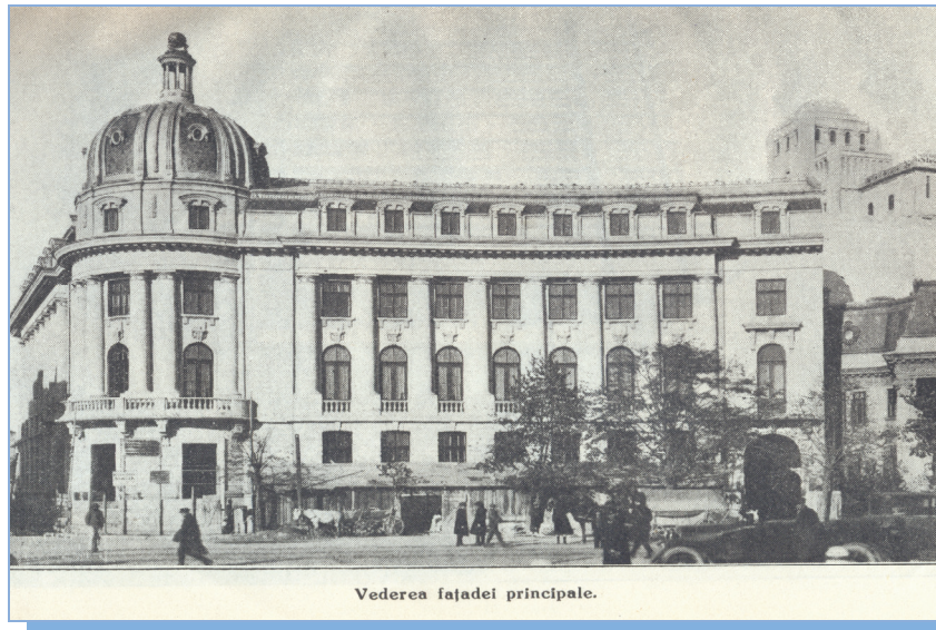
The Palace of the Bucharest University of Economic Studies, building completed in 1926
