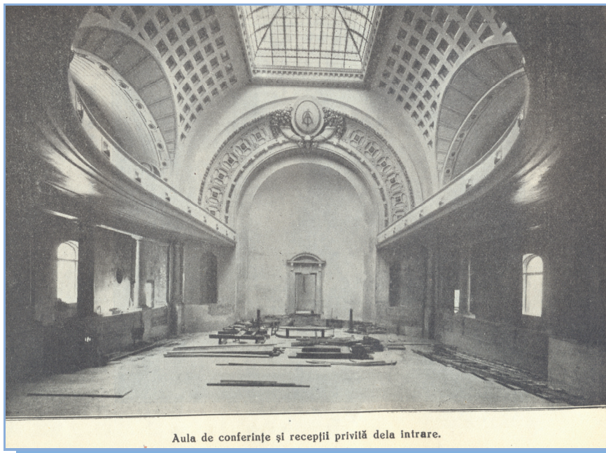
An entrance view of the Aula Magna, while being built
